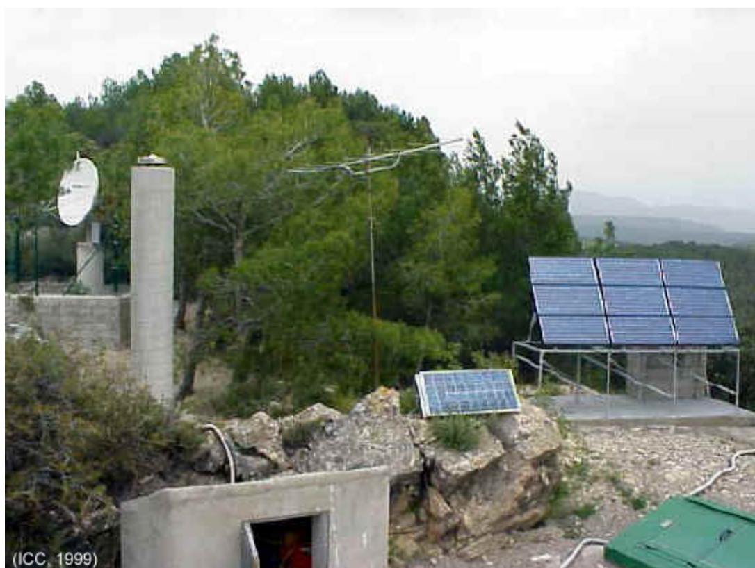
General view of the diferent elements: VSAT antenna, old telemetry antenna, geodetic pillar and GPS antenna at
