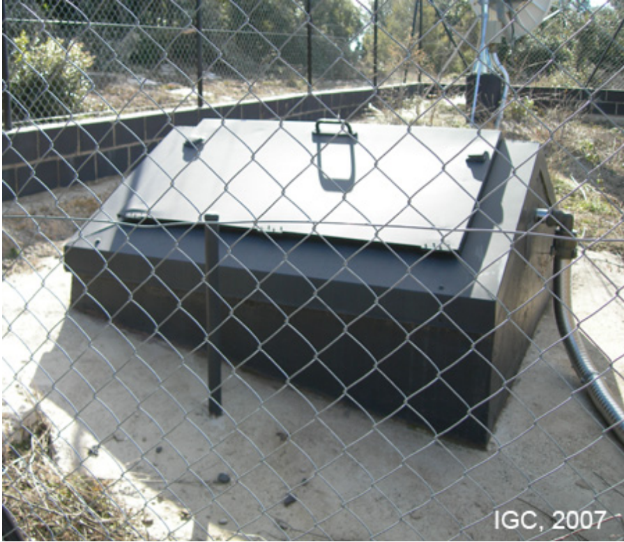
View in detail of the seismic vault at the surface.
