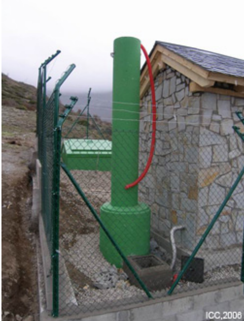
View in detail of the geodetic pillar and fence
