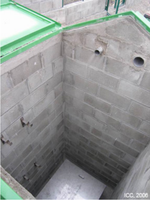
View in detail of the seismic vault
