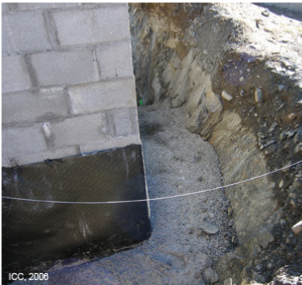
Geologic conditions: Rocky outcrop (pelites, grainstones and graywacke, Paleozoic).
