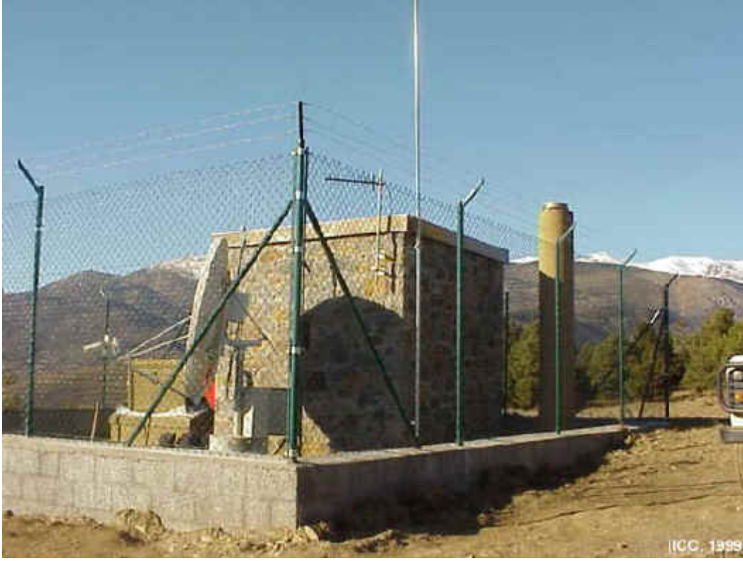
Back side view of the instrumental house where you can see the VSAT antenna and the GPS antenna at the top of the geodetic pillar.
