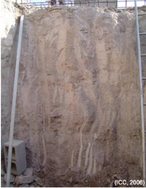
Geologic conditons: Rocky outcrop (grainstones with glauconite, Paleogene).
